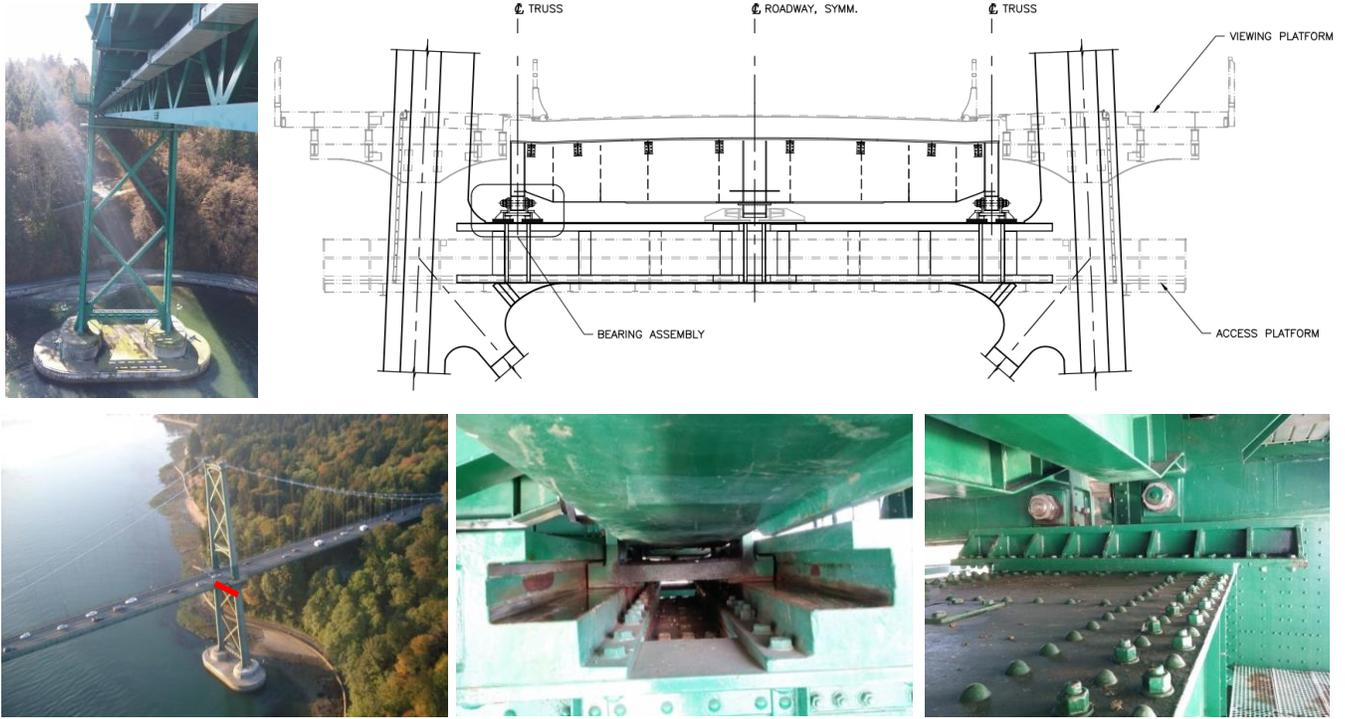
Figure 2. Clockwise from bottom left: Aerial view of south tower with tower strut highlighted in red; view of south tower from below deck; view of tower segment from drawings showing tower strut deck diaphragm, truss bearings; bearings within bearing guides supported on top of tower strut; previous deteriorated bearing shoe within bearing guides.
